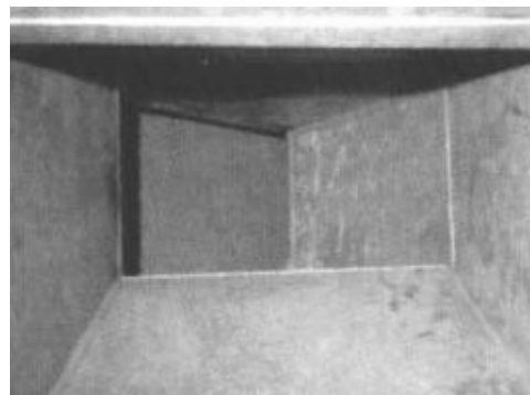
The duct after cleaning.
